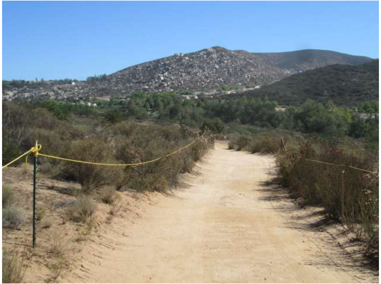
Photo 8: Environmentally Sensitive Areas were roped off along access roads to ensure construction crews avoided these areas (MM-CUL-1).
