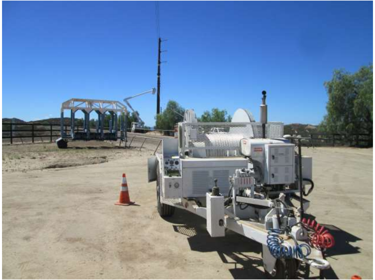
Photo 4: Fiber optic wire pulling at Stringing Site 13.
