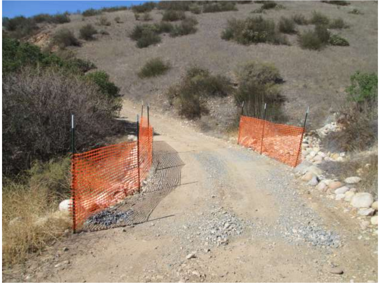
Photo 7: Between pole sites P32 and D34, temporary orange fencing used to guide vehicles away from the road ledge and preserve integrity of an adjacent drainage was observed intact and functional (APM-HYD-1).
